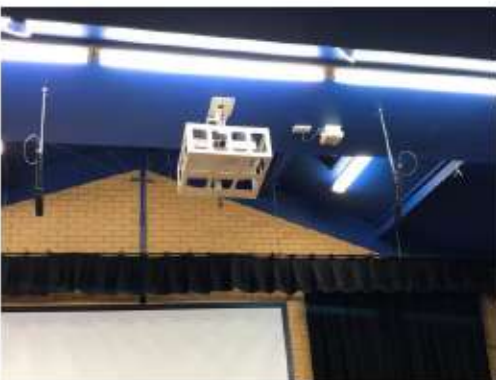
Stage Microphones mounted on the Stage Roof
